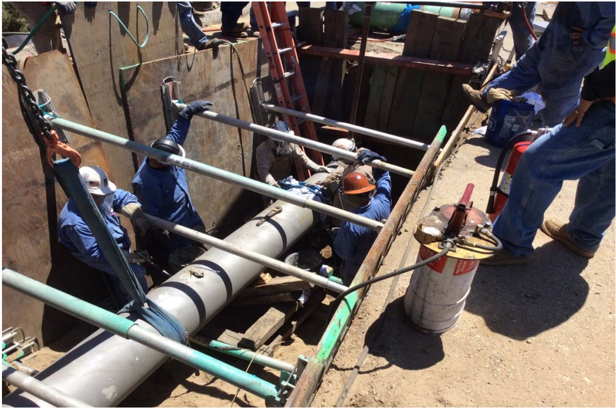
Figure 19: Section 2A Cut and Cap Activities
