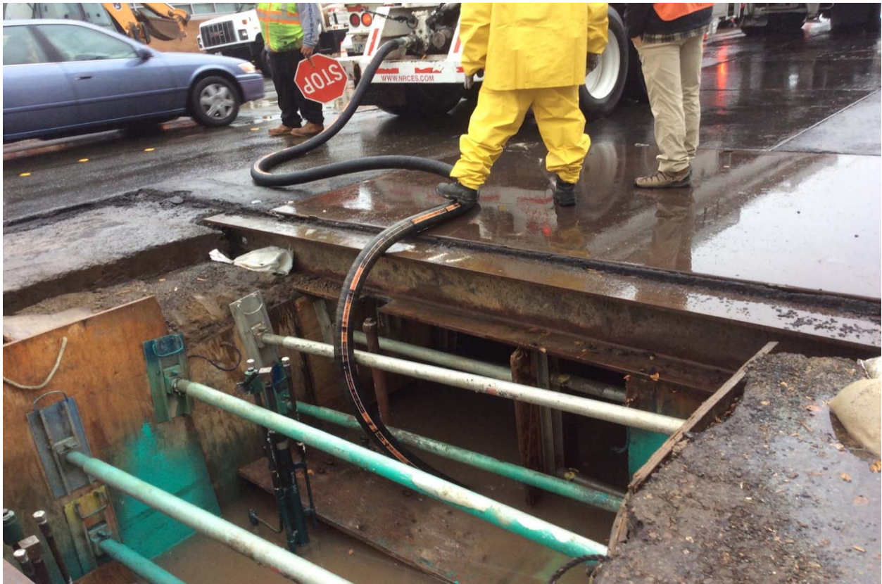
Figure 10: Pumping Water from Bellhole
