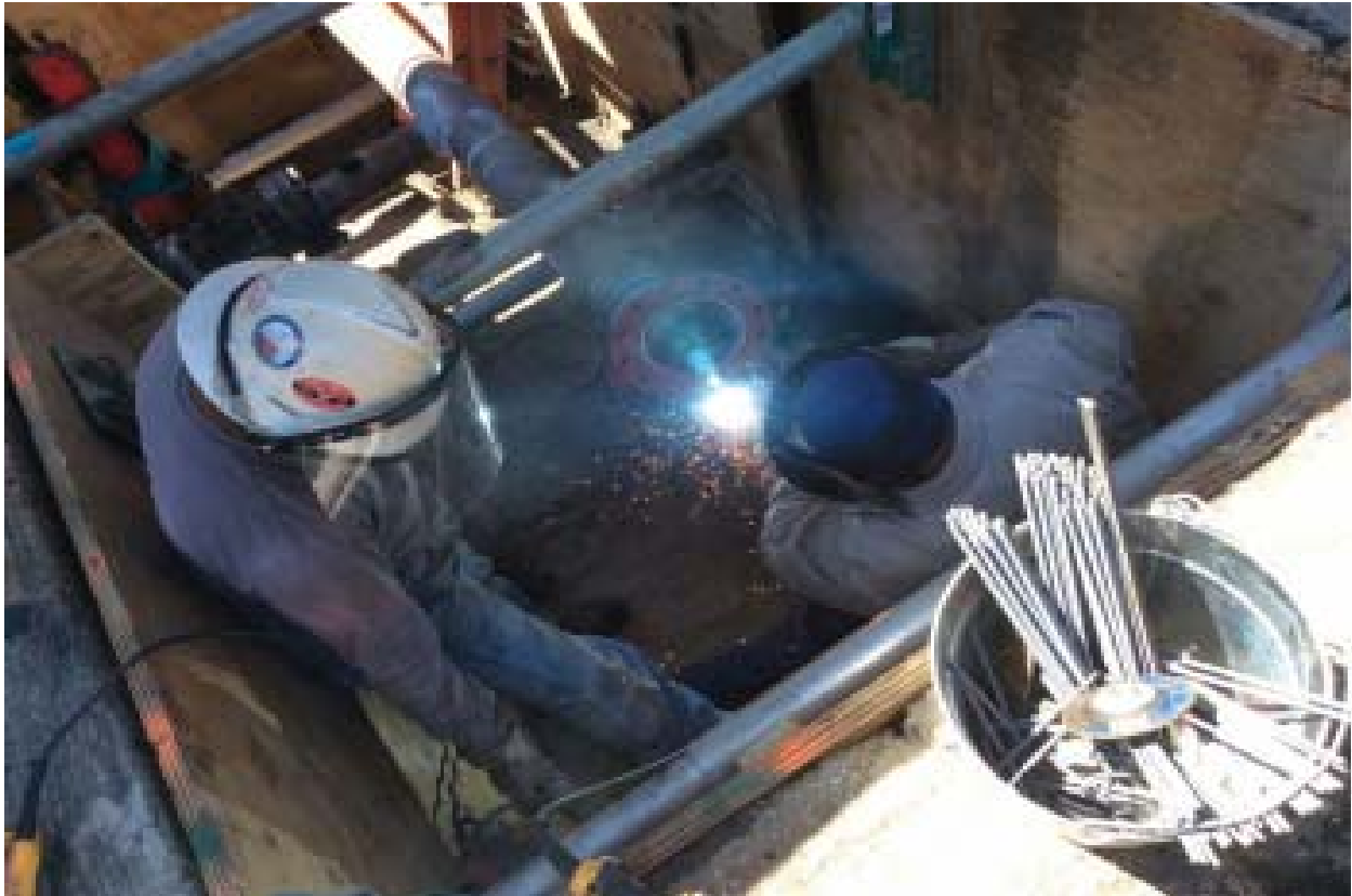
Figure 7: Installation of a Bottom Out Fitting
