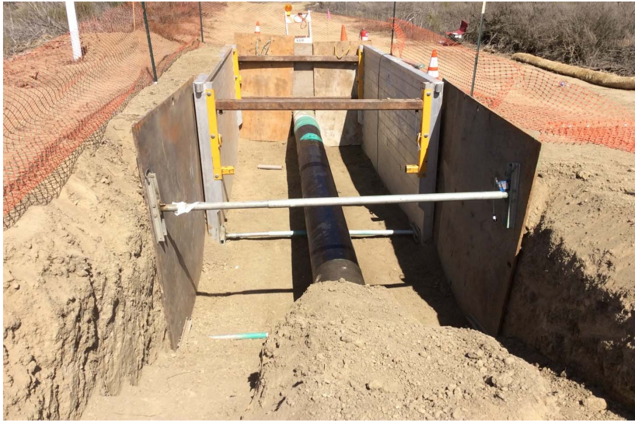
Figure 17: Section 2 West Tie-in Piece Along Hill Side
