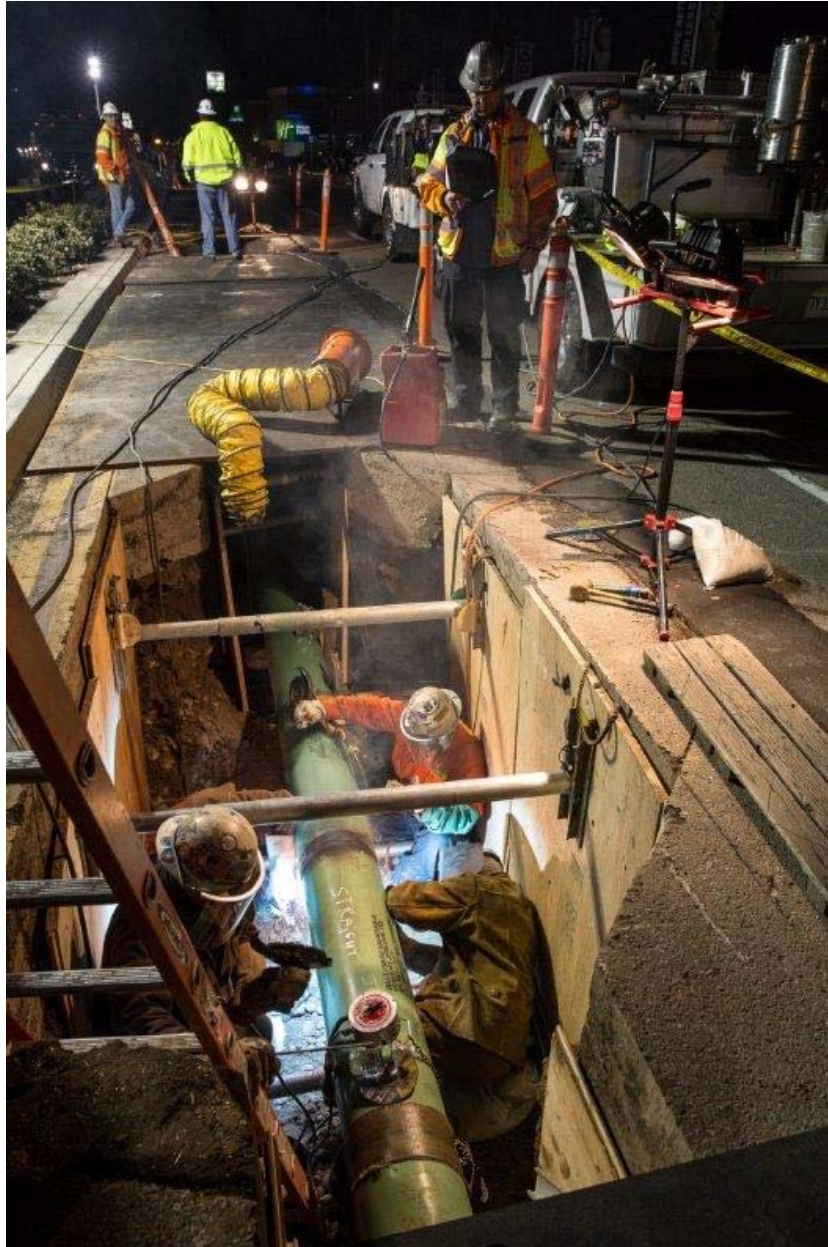
Figure 8: Night Work on Mission Bay Drive
