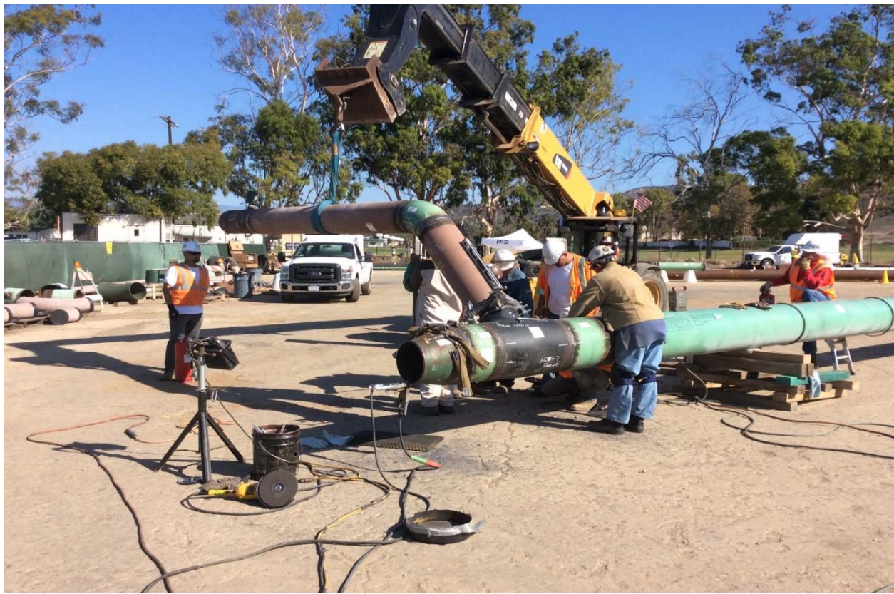
Figure 15: Section 1 Pre-fabrication of Replacement Pipe
