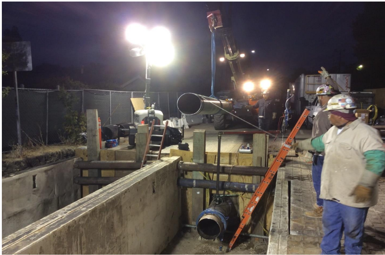
Figure 7: Crew Lowering Tie-in Piece at Burbank Boulevard
