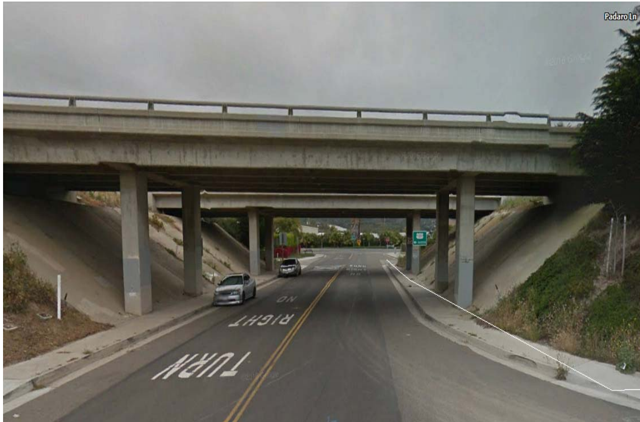
Figure 7: Underpass Site of New Crossover Line 8119
