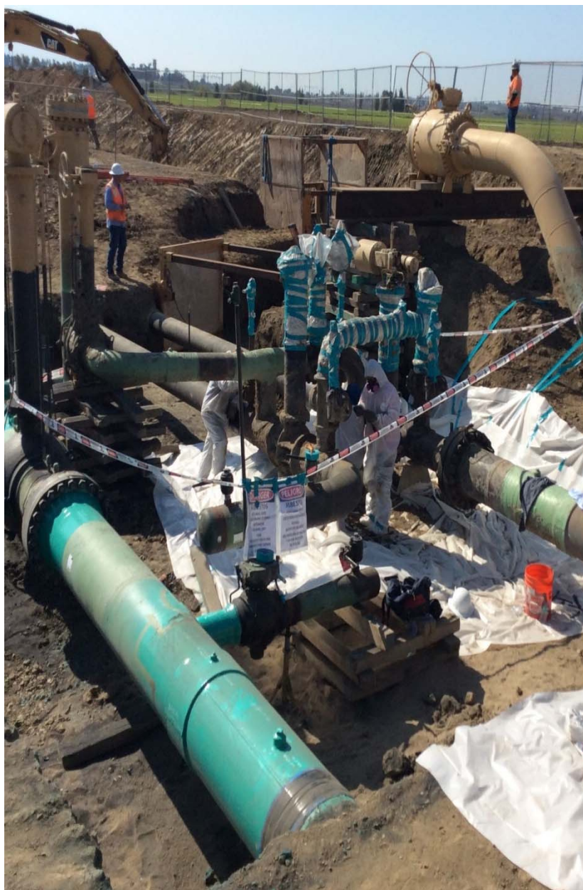
Figure 23: Section 3A Abatement Activities of MLV Removal
