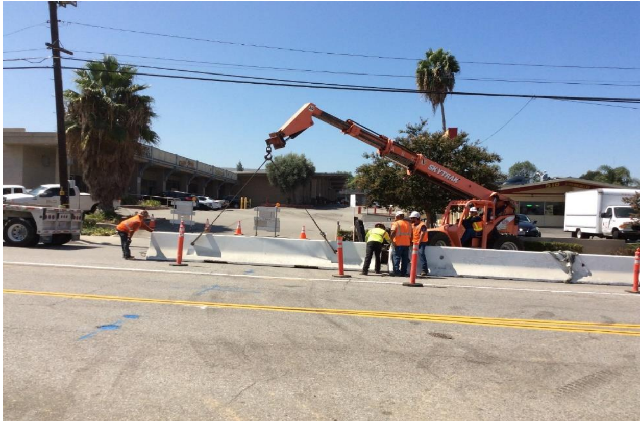
Figure 3: K-Rail Set Up Along Don Julian Road
