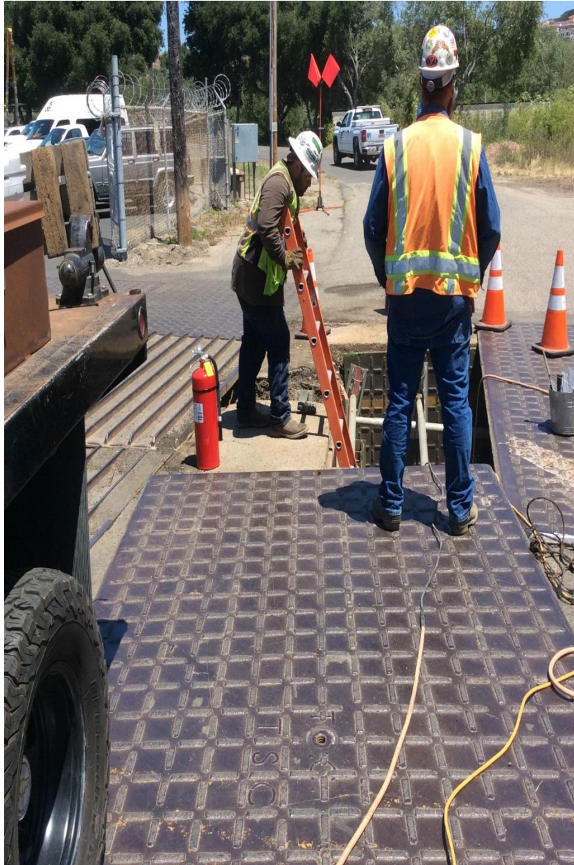
Figure 4: Setting up to Weld on Bello Street
