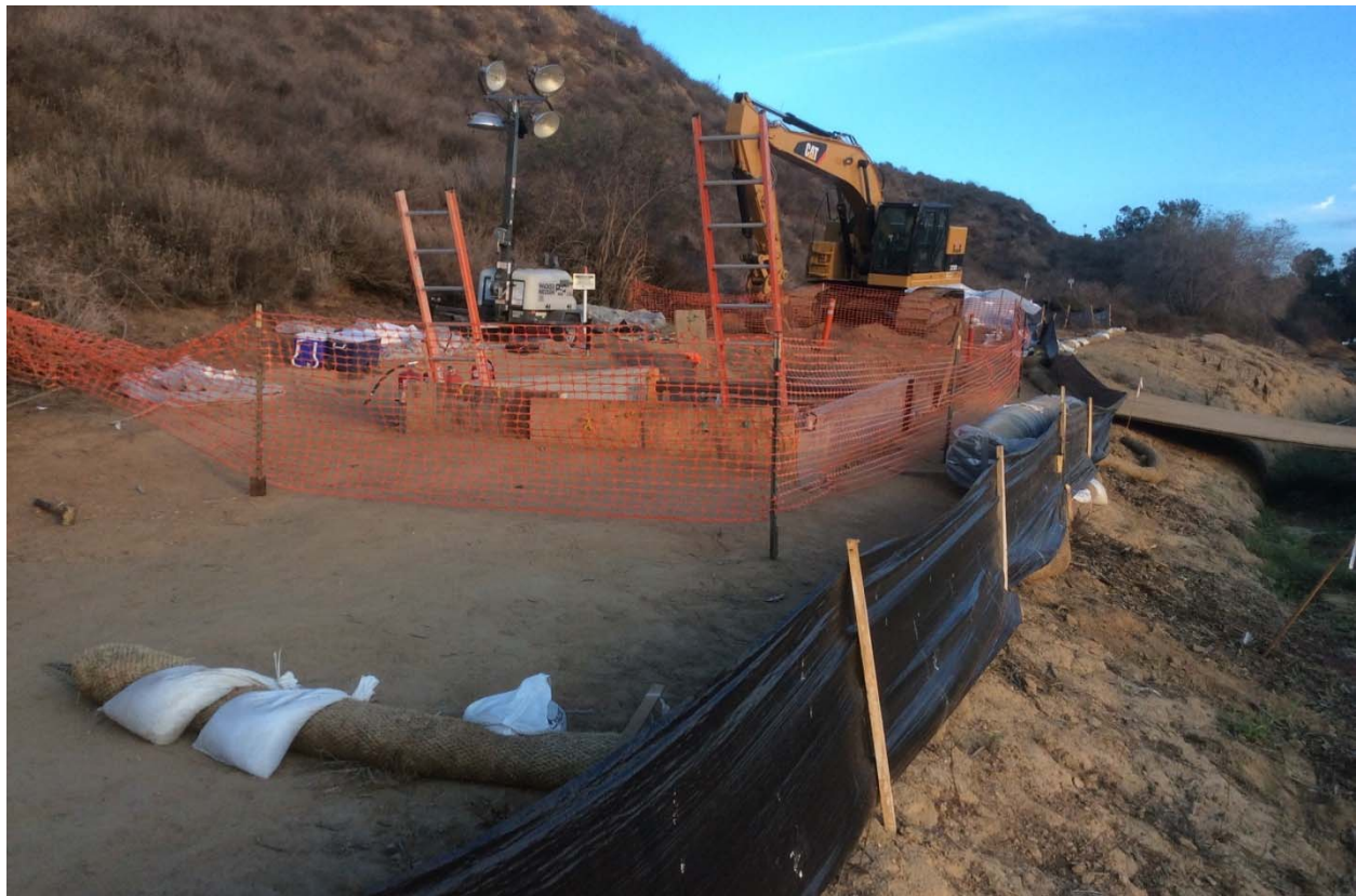
Figure 24: Section 4 and 5 West End Test Head Excavation
